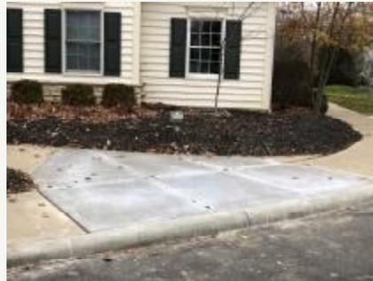
Parking lot curbs were fixed and the old handicap ramp removed on November 30. This work needs to precede resurfacing the parking lot in the spring.
