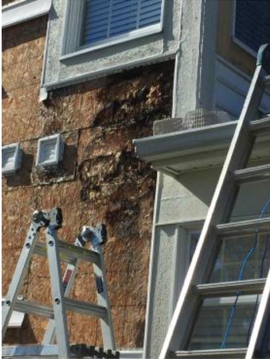
sheeting and applied Tvek to the area affected. He could literally push his finger through the damaged OSB. We are hopeful that the damage has not penetrated the studs which will be considerable added cost to the repair.
