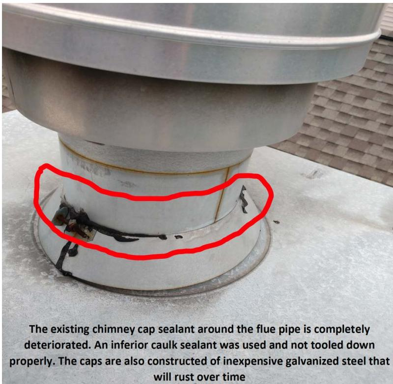
**The existing chimney cap sealant around the flue pipe is completely deteriorated. An inferior caulk sealant was used and not tooled down properly. The caps are also constructed of inexpensive galvanized steel that will rust over time**
