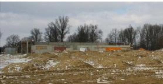
The re-enforced concrete roof will be constructed after the weather warms and the supporting side and internal structure work is complete.
